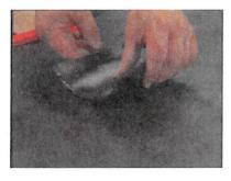
**Step 4**- Install the QuickSeam patch by peeling away the release paper and placing the patch over the damaged area of the liner.
