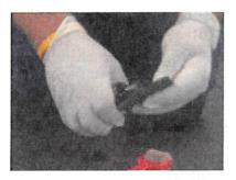
**Step 2**- Apply the QuickPrime™ Plus Primer by pouring a small amount onto the scrubber pad and applying it to the surface of the PondGard panel beyond the perimeter of the area to be repaired with a patch.
