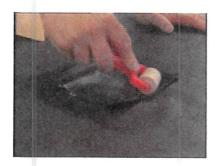
**Step 5**- Roll the patch evenly over the area to be repaired in order to properly mate the patch and liner together.
